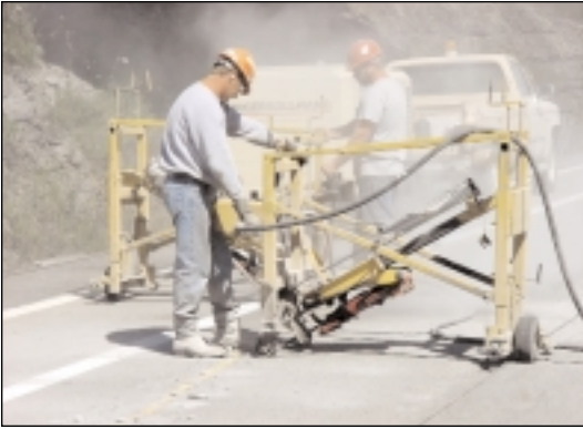
1. Drilling hole for tiebar along longitudinal crack using frame-mounted drill rigs.
