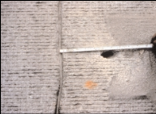
3. Checking hole location.
