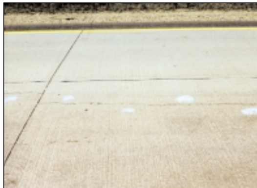
6. Completed cross-stitching on longitudinal crack.
