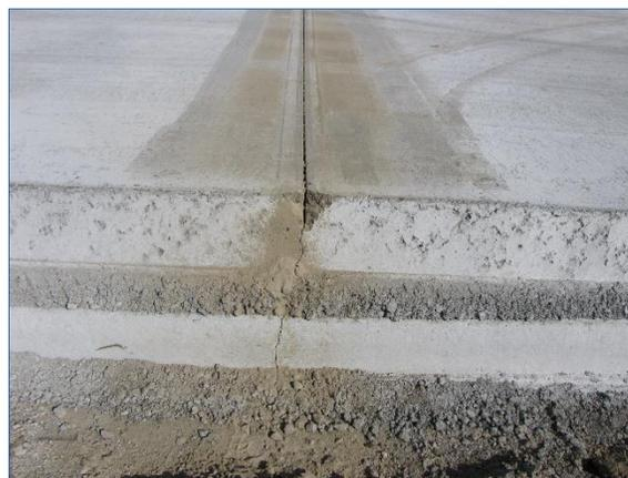
*(Right) Photo shows close-up of a sawcut on the new pavement.*
