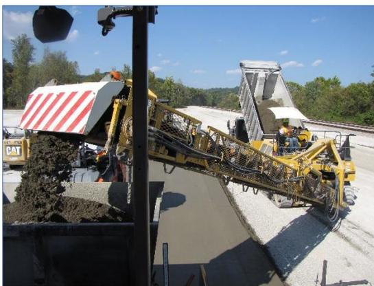
*(Above) Concrete is deposited to the placer component ahead of the paver.*
