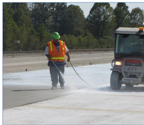
*(Top right) Equipment operator applies curing compound.*
