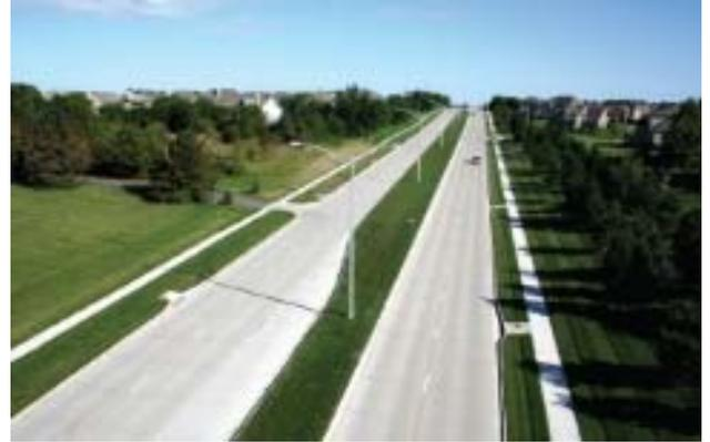
*Reconstruction of Nall Avenue between 143rd and 159th in Leawood and Overland Park, Kansas, involved building a new roadway using 9-in. thick concrete across 4 lanes.*
